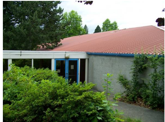
Main building (306A), south (rear) elevation at enclosed corridor between the Holladay Center and Youngson School, looking northwest.
