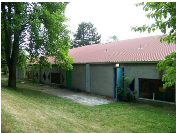
Main building (306A), east (side) elevation, looking southwest.
