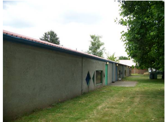
Main building (306A), west (side) elevation, looking south.
