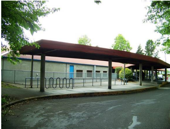
Main building (306A), north (front) elevation, looking southwest.
